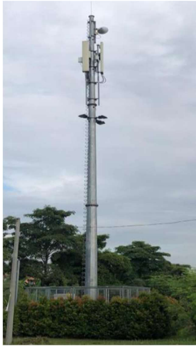
Figure 5. Steel monopole
