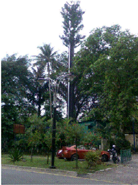
Figure 13(a). Site 1 - View 1 (Overall)
