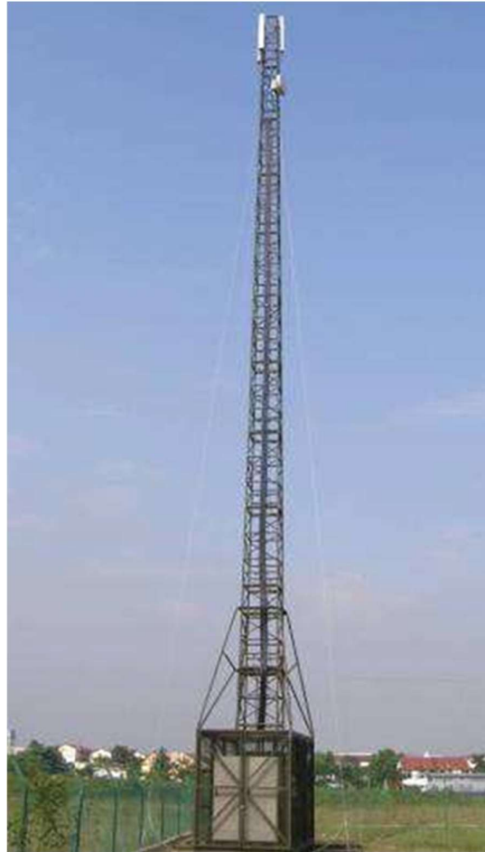
Figure 16. Portable BTS
