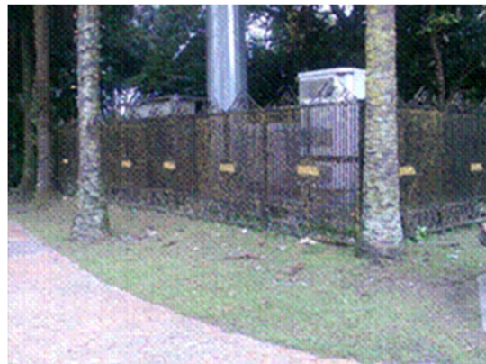
Figure 13(d). Site 2 - View 2 (Close-look)
