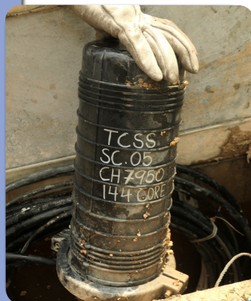
Picture 2: Holes for fibre optic cables and fixed links on the West Coast Expressway (WCE)
