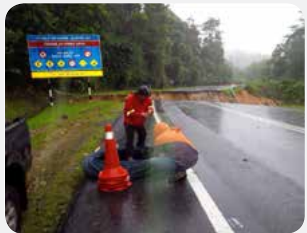
Reinstalling disconnected fibre cable due to landslide
