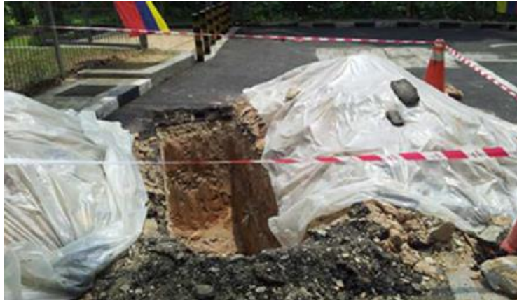
Figure 3. Site preparation (starting hole)
