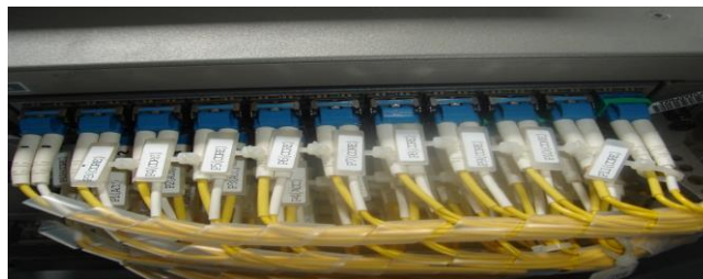
Figure 51. Sample of recommended tagging system
