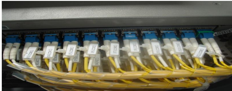
Figure 62. Sample of recommended tagging system
