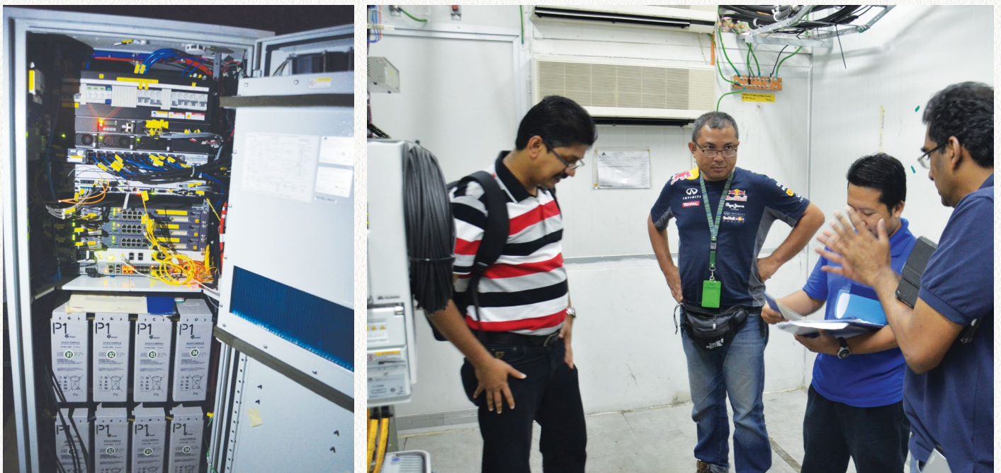
Site visit involving AA inspection, compliance verification and trial transmission
