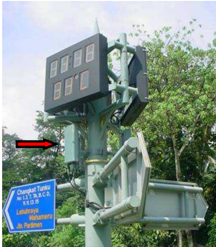
Figure 3. Arrow shows a panel antenna on a signage pole with clock (multi-purpose). The antennas go unnoticed among the signages.
