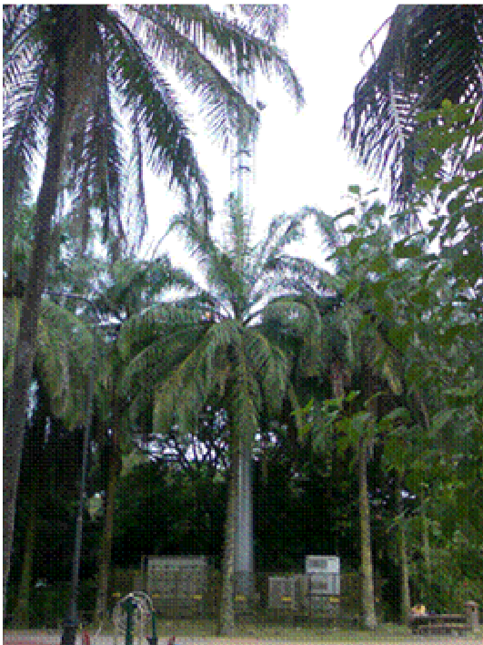
Figure 6.3 Site 2 - View 1 (Overall)
