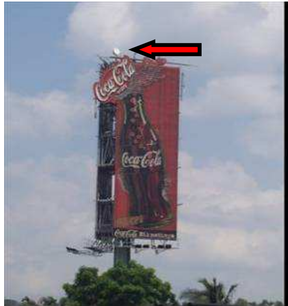
Figure 9. Antenna on top of structure
