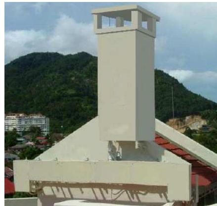
Figure 11. Chimney Concealment System
