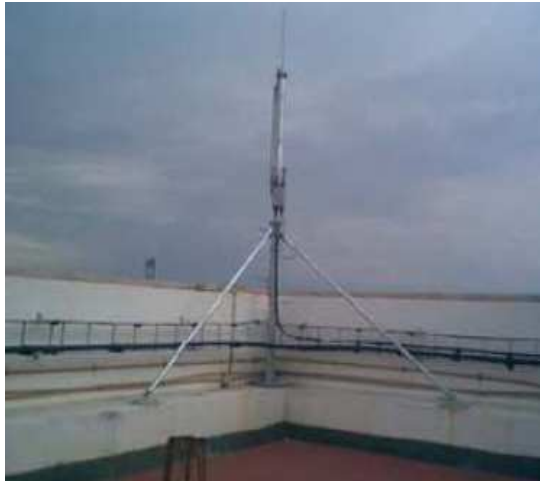
Figure E4. Examples of RoofTop Outdoor with 3m/6m Poles
