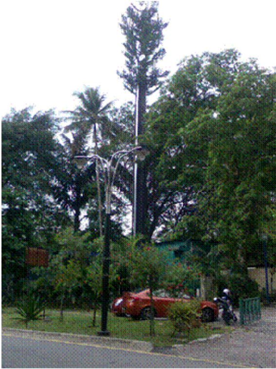
Figure 6.1 Site 1 - View 1 (Overall)
