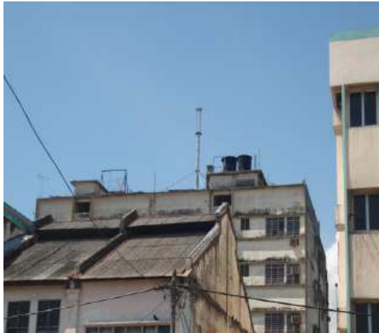
Figure E6. Examples of RoofTop Outdoor with Unipole
