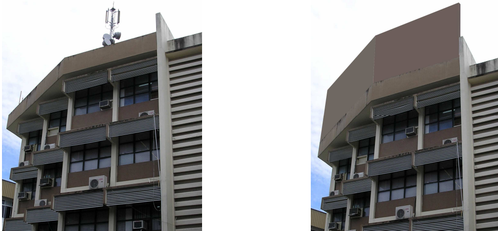
Figure 13. Roof Top Concealments
