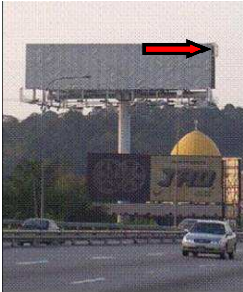
Figure 8. Highest mountable point on the structure
