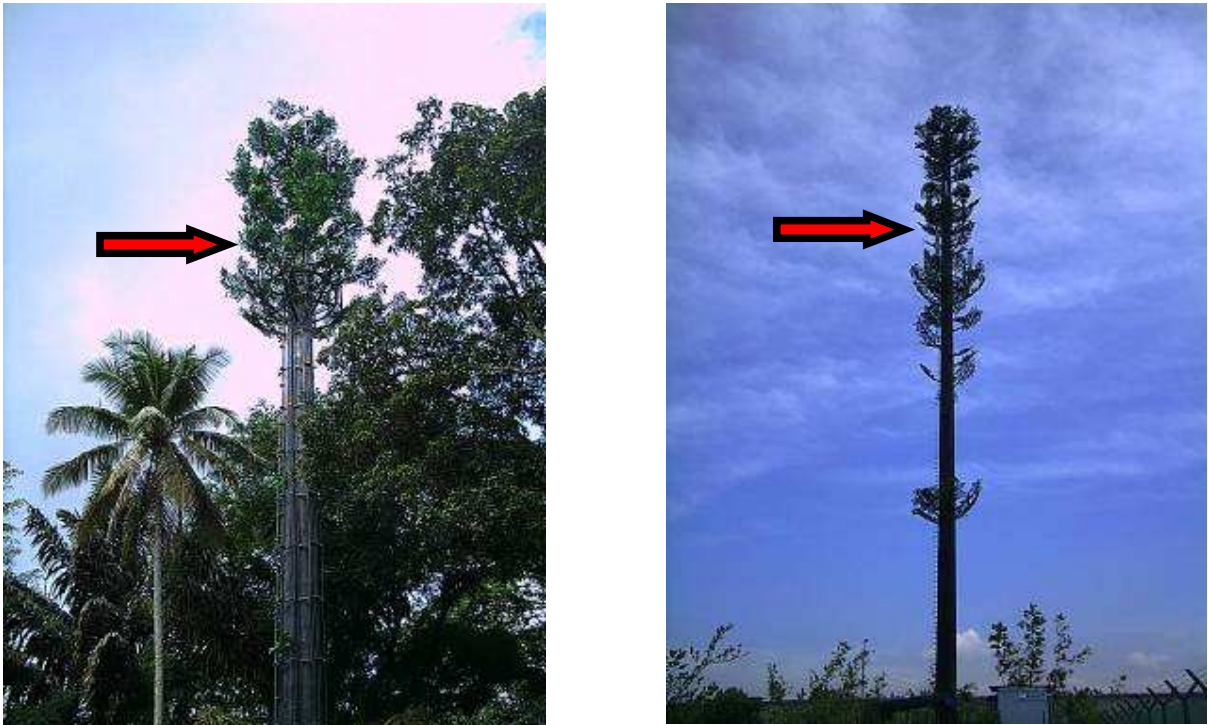
Figure 2. Arrows in the pictures above indicating the antennas which are installed under the cover of the artificial foliage.
